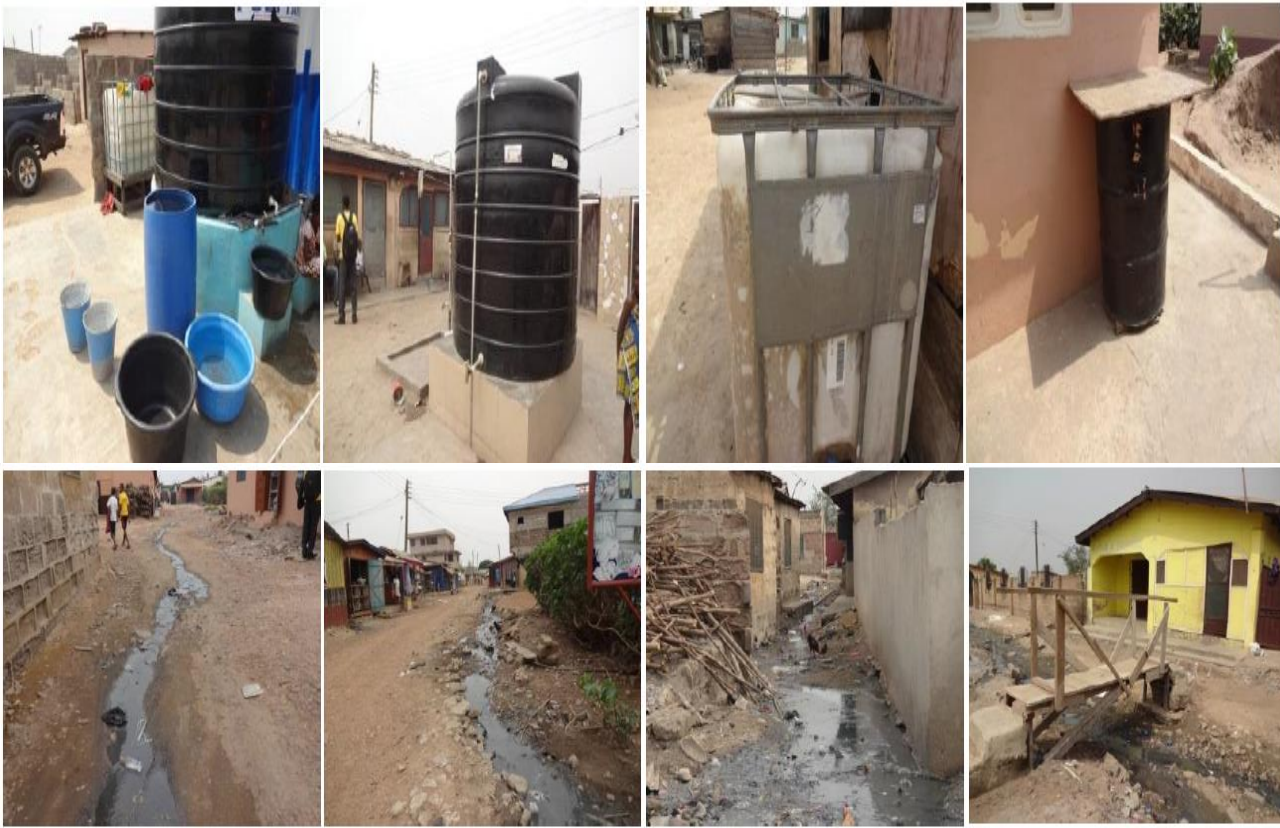
Plate 7.3: Evidence of poor drainage (lack of stormwater and sullage drains) situation in some parts of the community
